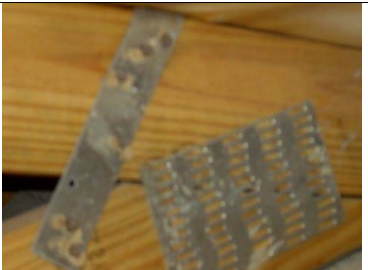
Roof to wall attachment
